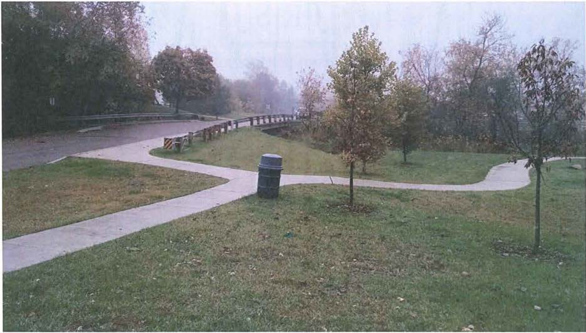
Willowbrook Drive Bridge Rehab and New Pathway along Willowbrook Drive and connection to Brookfarm Park Pathway
