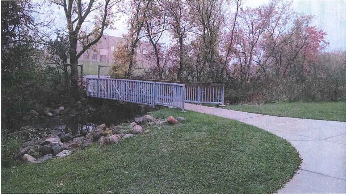
Newly replaced pedestrian bridge connecting Brookfarm Park to Village Oaks Elementary.
