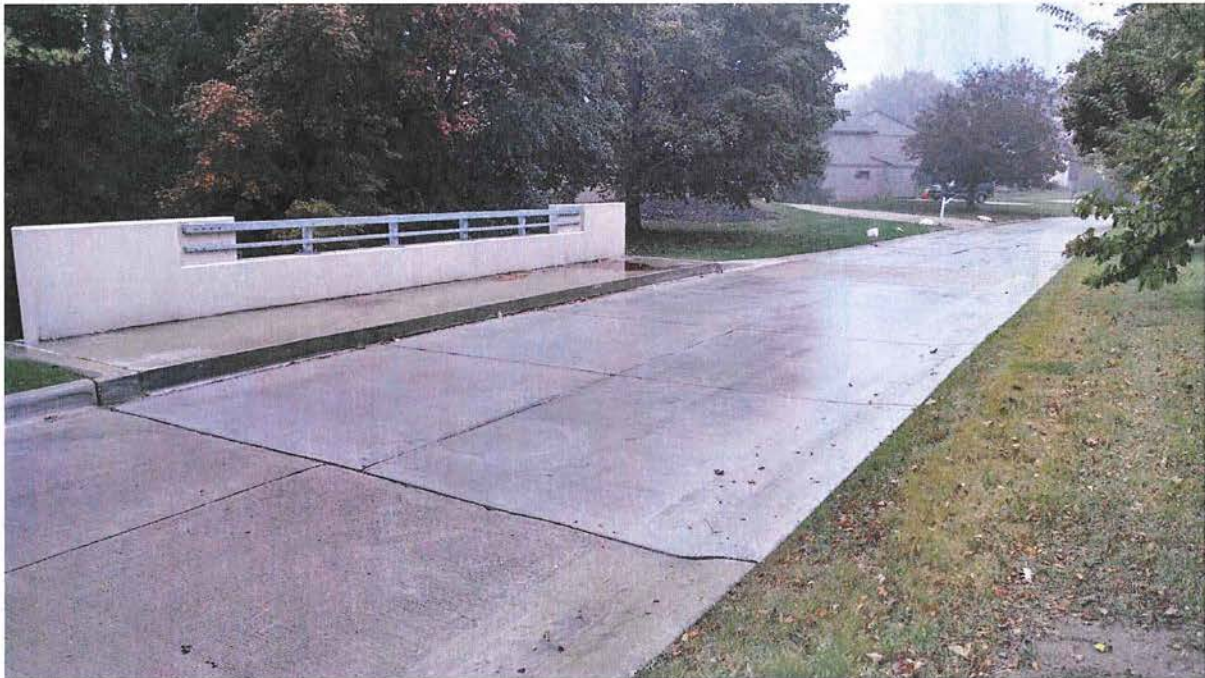
Rehabilitated Cranbrooke Drive Bridge over Ingersol Creek.
