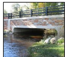
Figure 4: Three-sided box bridge
