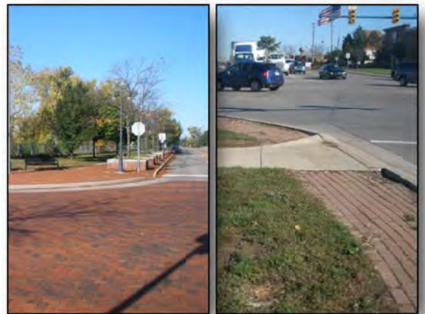
Large expanses of brick paving should be avoided due to maintenance issues. Instead, brick should be used as an accent to a concrete walk or plaza.
