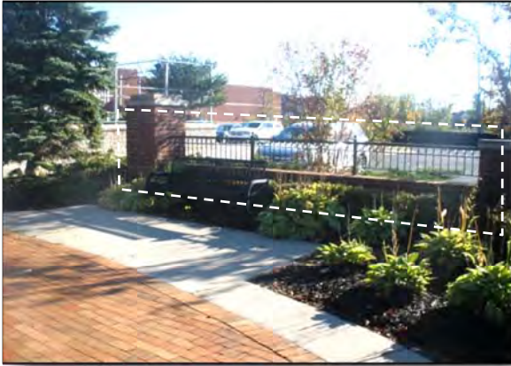
Encourage use of a low, masonry wall and column with metal fence combination, as shown in Main Street area.
