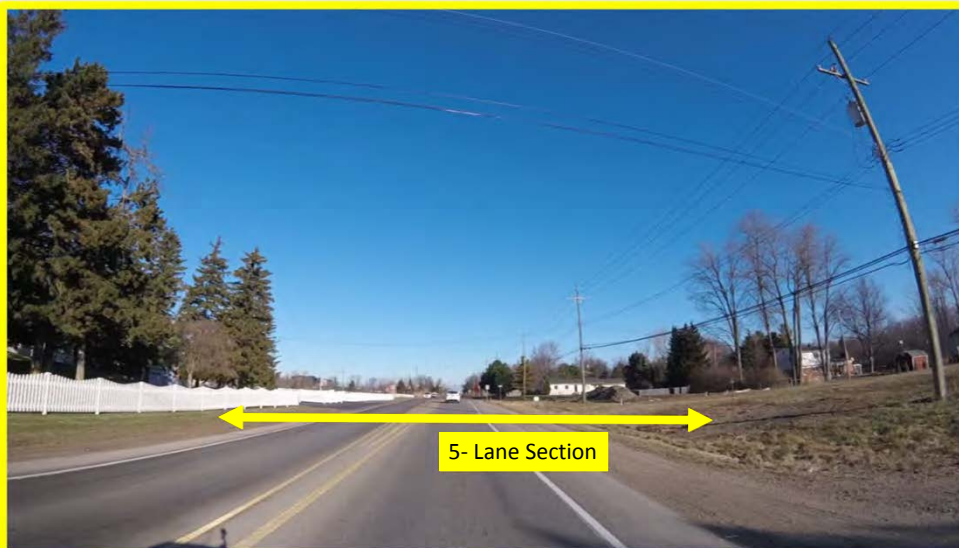
Northbound Beck Road, South of Eleven Mile Road
