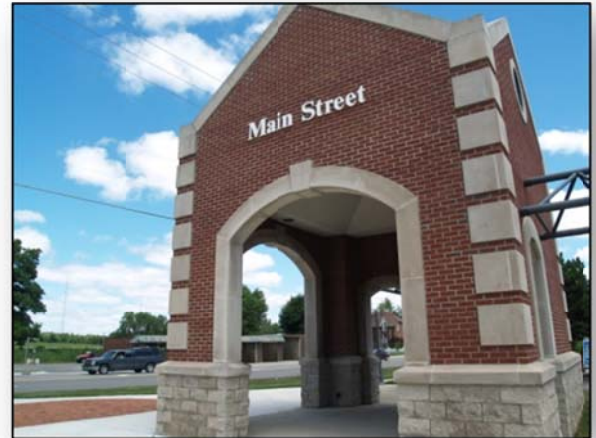
Existing entry structure provides opportunity for pedestrian connections to redevelopment.
