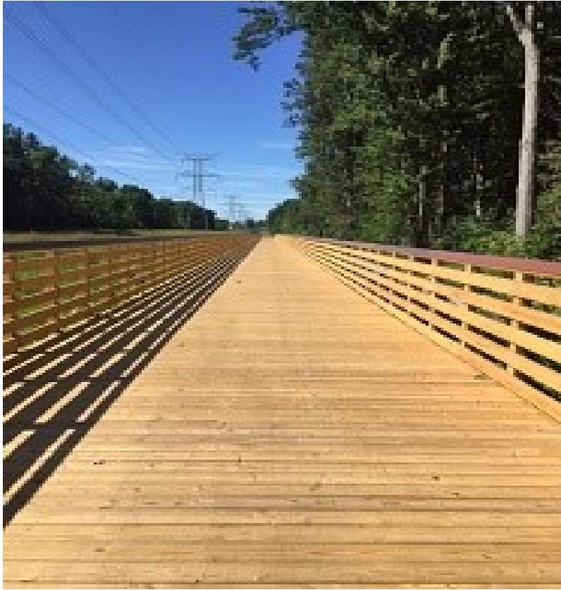
Close up of the 16-foot-wide boardwalk, just north of 9 Mile Road
