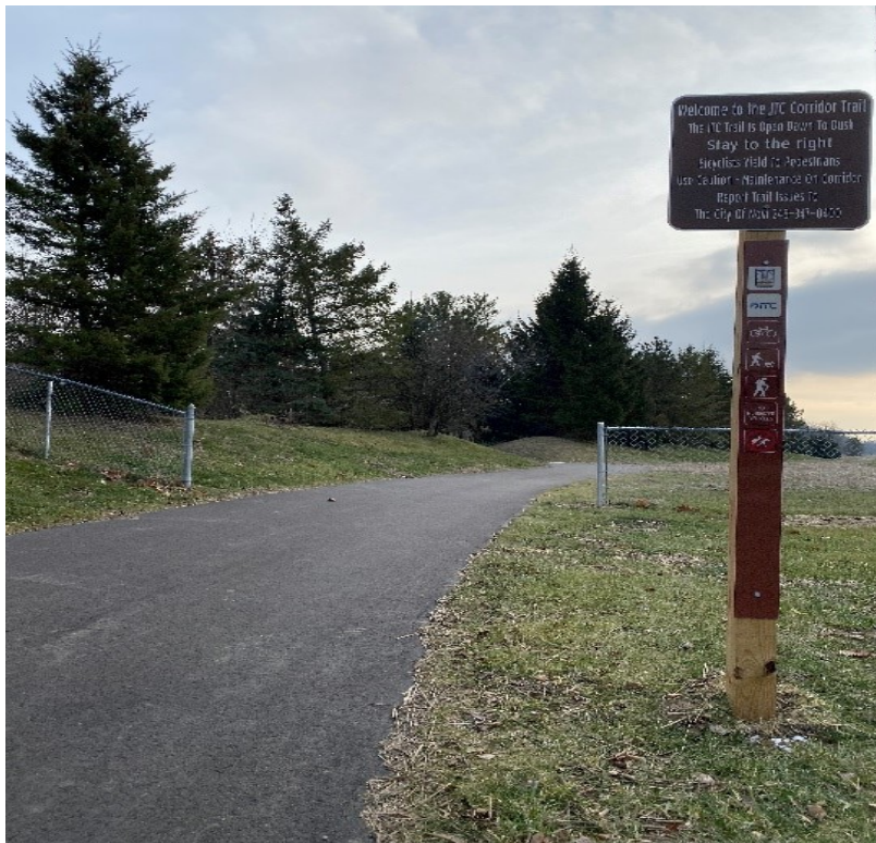
Installation of new wayfinding signage along the pathway (just south of 10 Mile Road)
