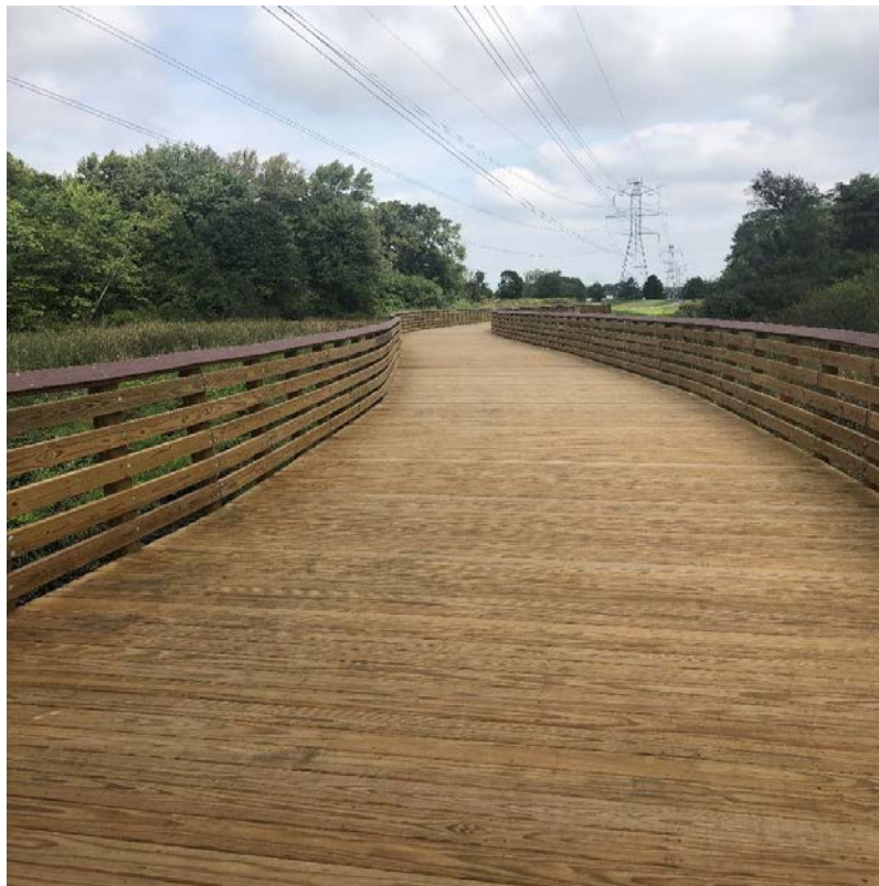
S-curve in the 16-foot-wide boardwalk between 9 and 10 Mile Roads
