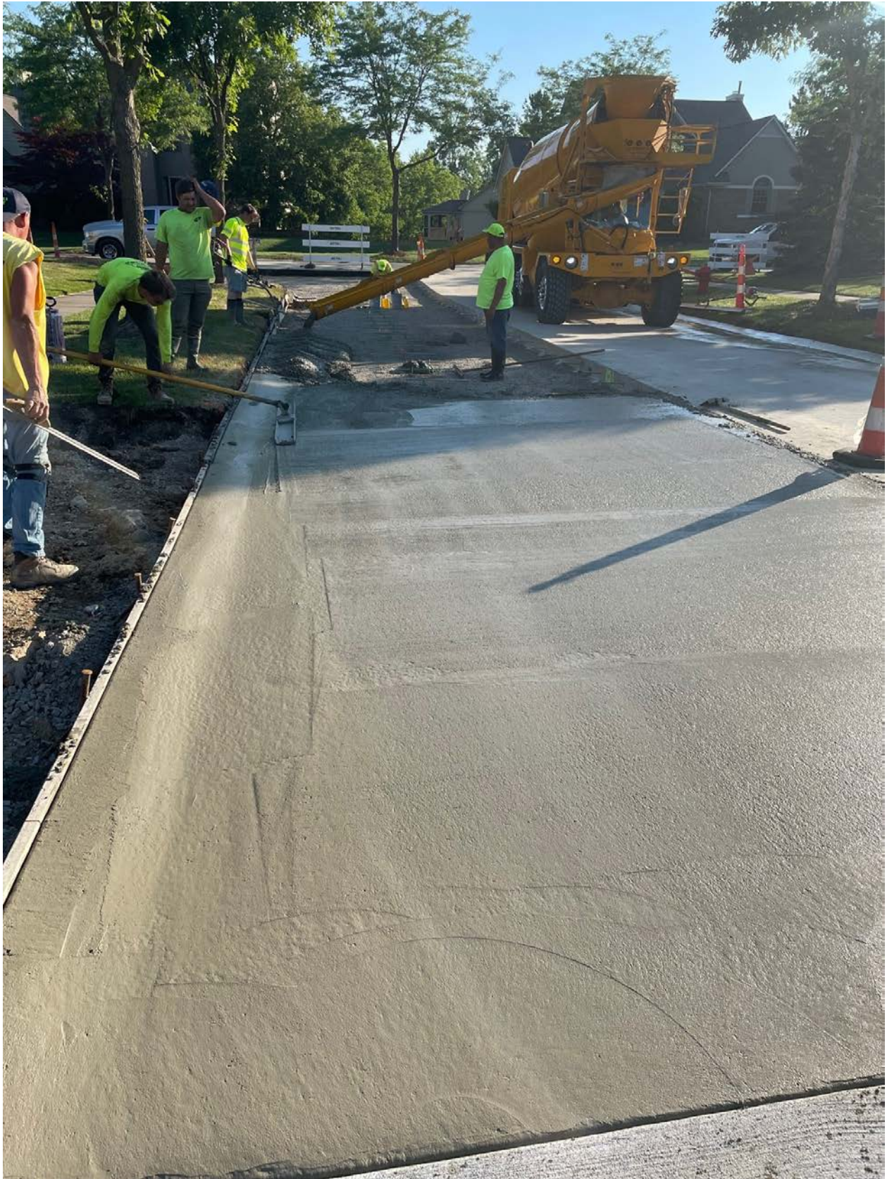
South Lake Drive (Bristol Corner Subdivision) – DURING construction
