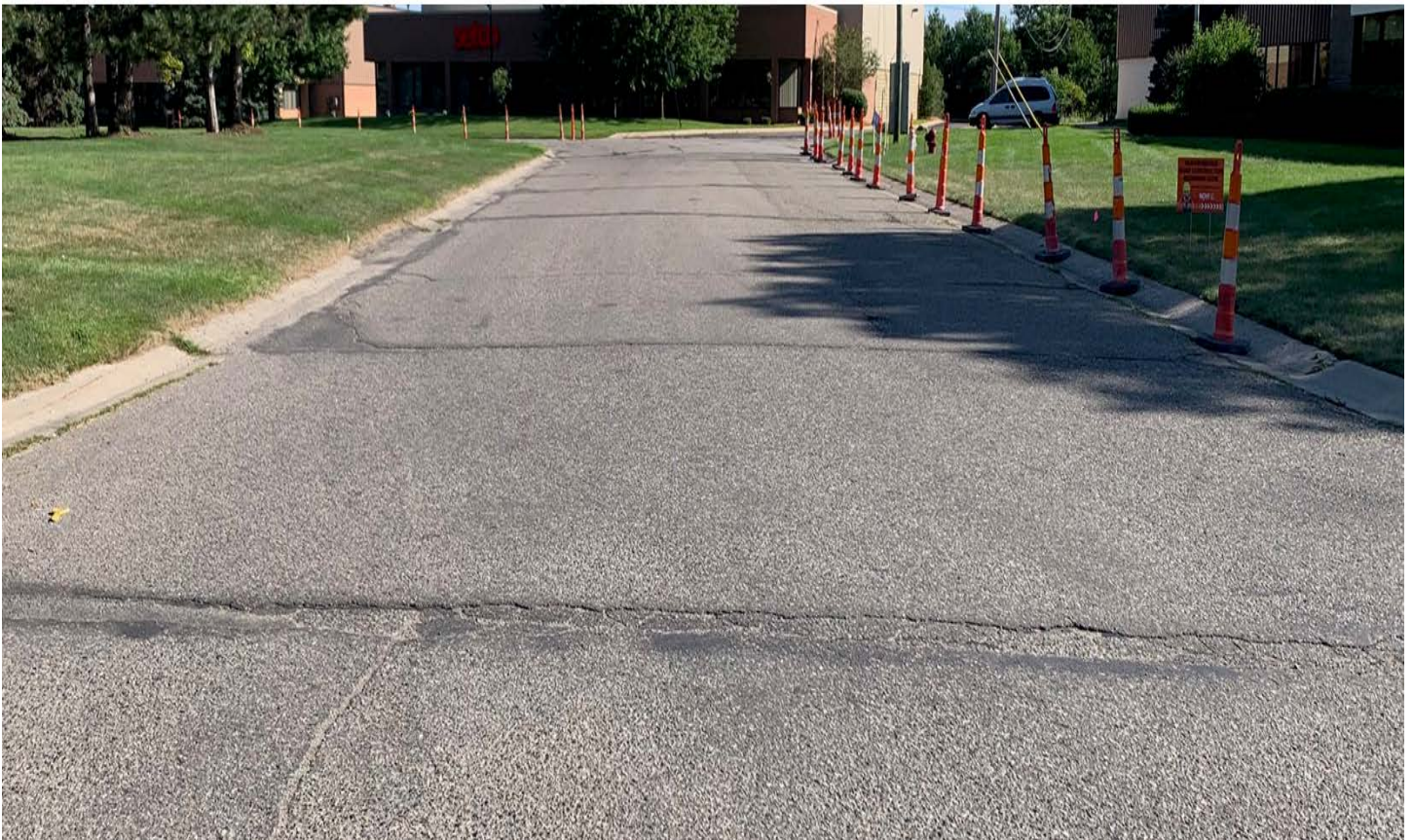
Jo Drive – Pre-Construction of asphalt roadway
