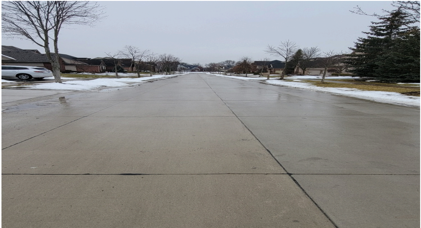
Sterling Drive (Bristol Corners Subdivision) – AFTER
