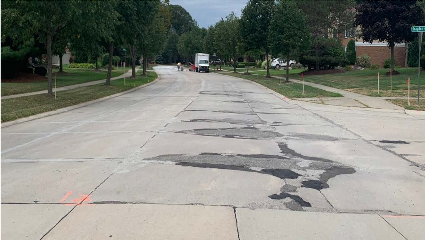
Royal Crown Estates – White Pines Drive – Pre-Construction
