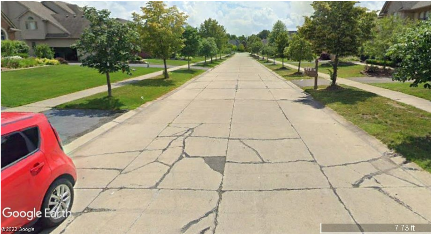
Sterling Drive (Bristol Corners Subdivision) – BEFORE
