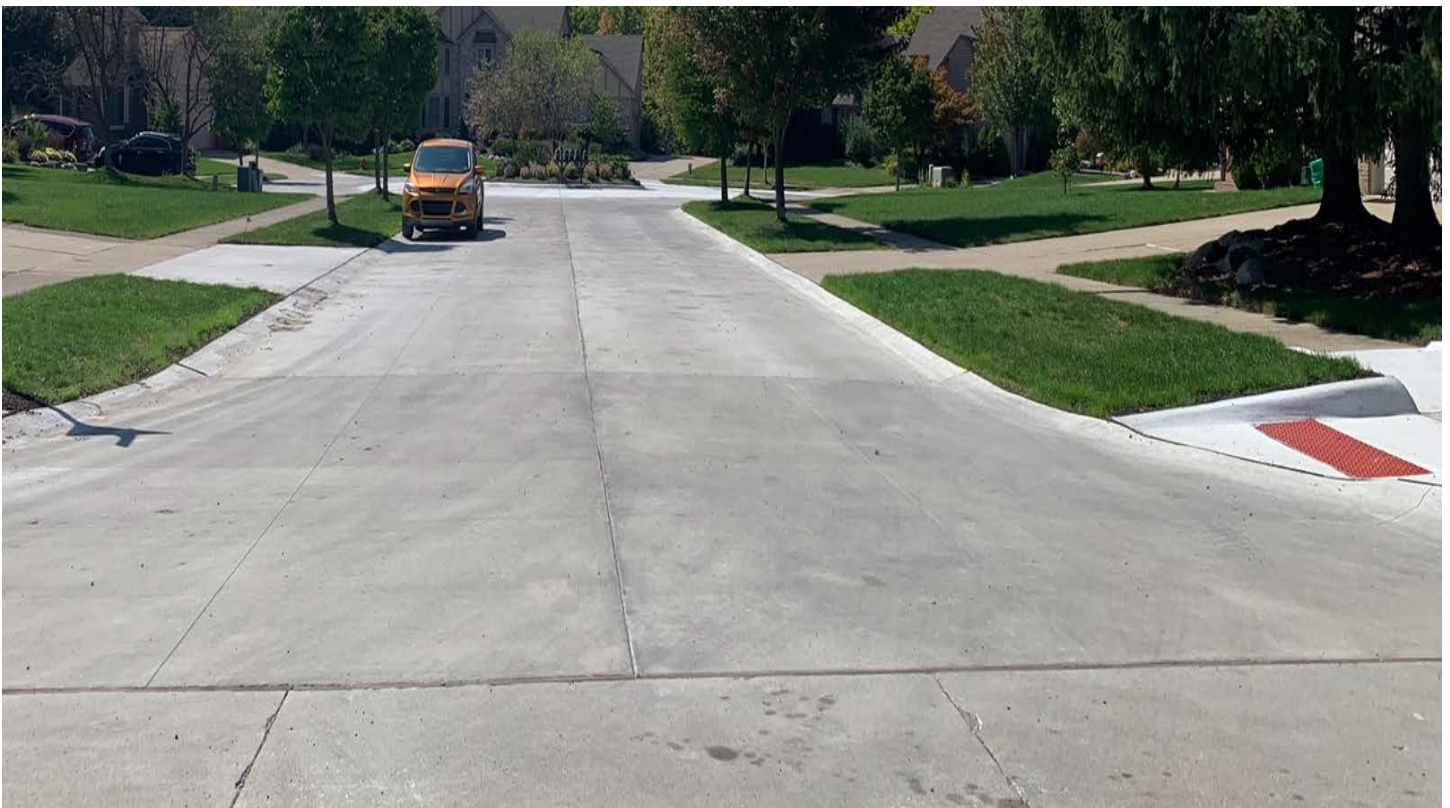
Cedarsprings Estates – Kerri Court – Construction completed and reopened
