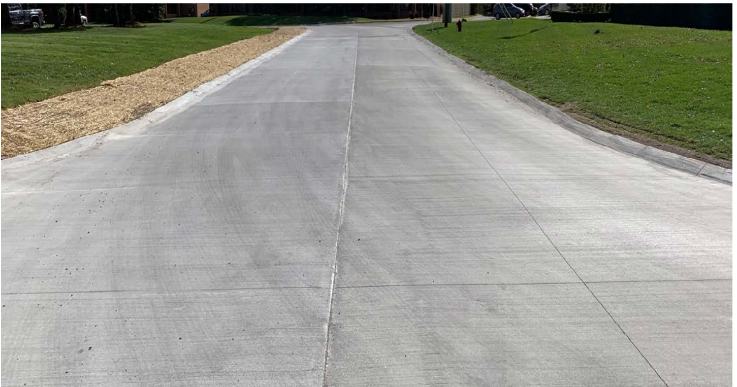
Jo Drive – Construction completed and reopened
