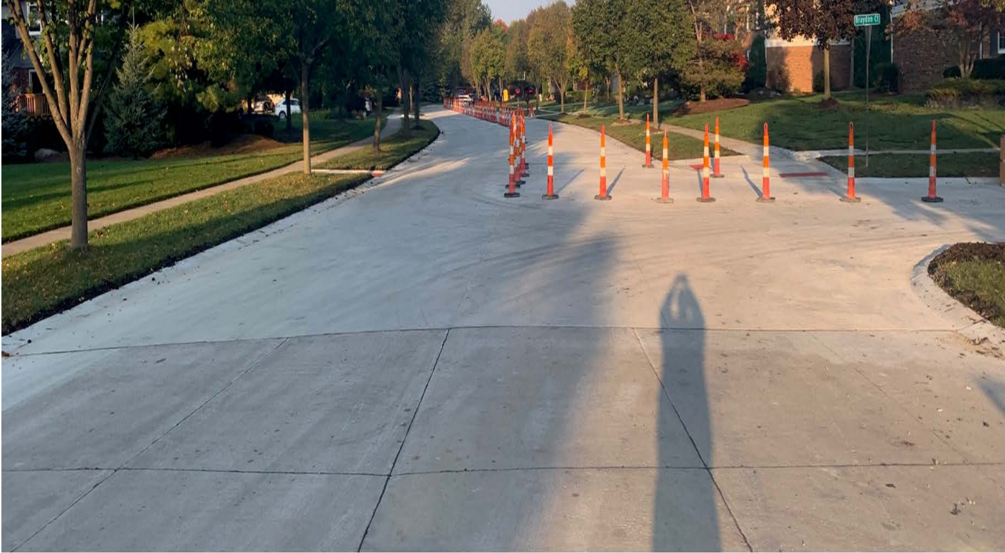
Royal Crown Estates – White Pines Drive – Completion of final concrete pour
