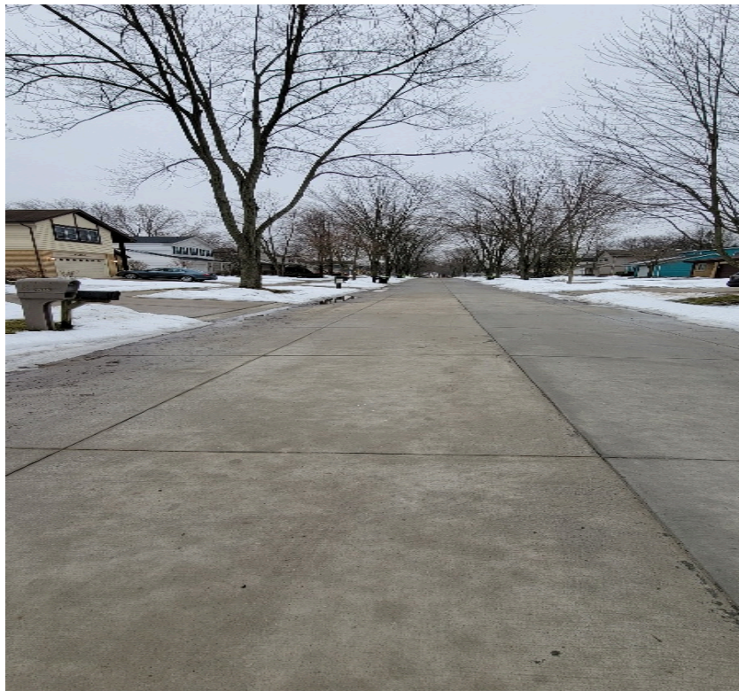
Park Ridge Road (Meadowbrook Glens Subdivision) – AFTER
