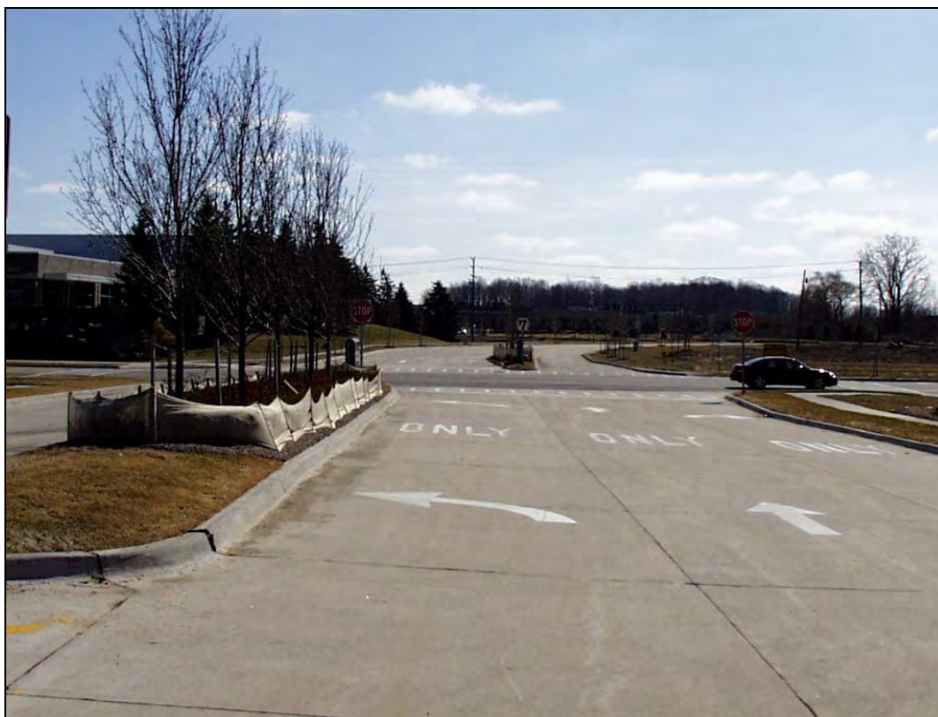
Figure 4. Cabot Drive at 13 Mile Road, Looking South
