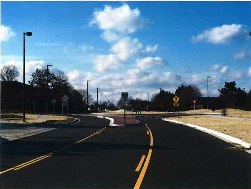
Crescent Boulevard – Looking east towards roundabout at Town Center Drive
