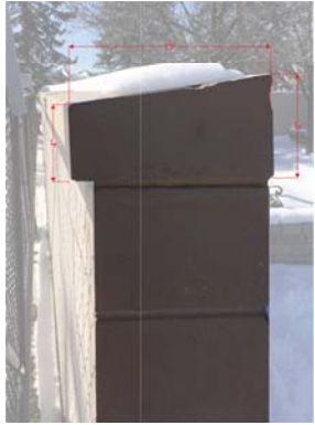
WALL CAP DETAIL (A) NOT TO SCALE
