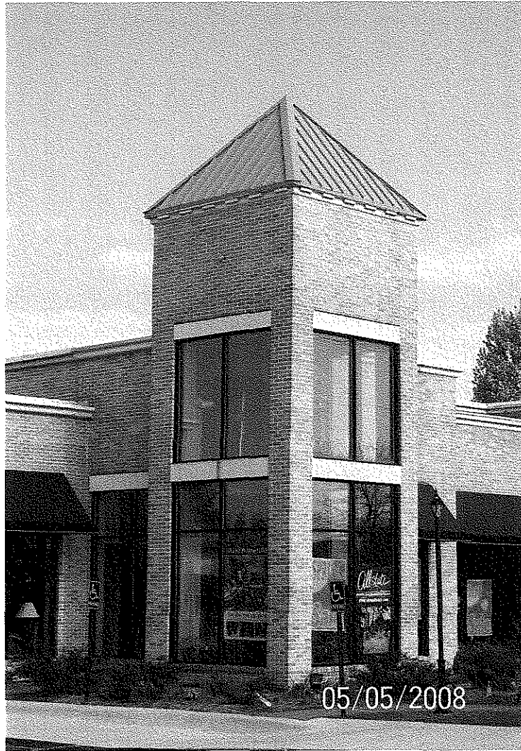
SHOWN IN THE PHOTO ABOVE THE SOUTH TOWER ELEVATION AND THE EAST TOWER ELEVATION ONE (1) WALL SIGN PROPOSED FOR EACH ELEVATION
