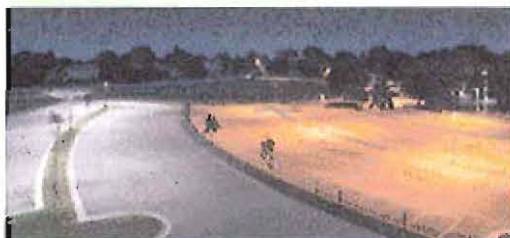
The parking lot lighting demonstration comparing LED (left) and high-pressure sodium (right) shows the even light distribution and good color rendering of LED lighting.
