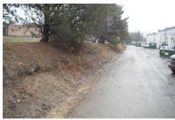
2. Rear of commercial center – Berm erosion; exposed meters, pipes, and Conduit; and unenclosed dumpsters
