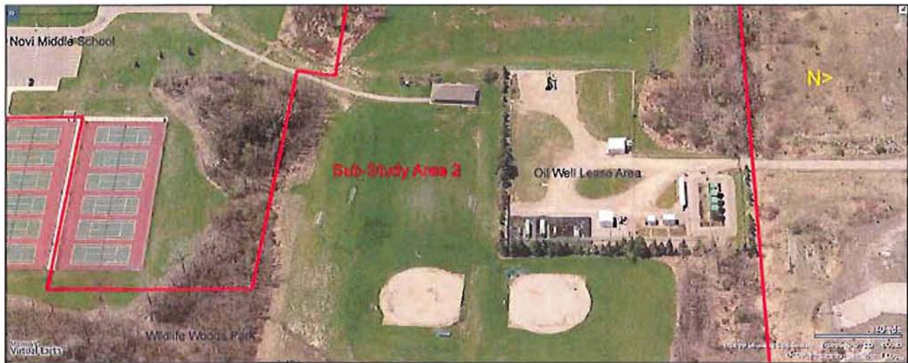
Figure 15 – North portion of Sub-Study Area 2 with oil facility looking west toward Wixom Road (source Microsoft Corp. 2009).
