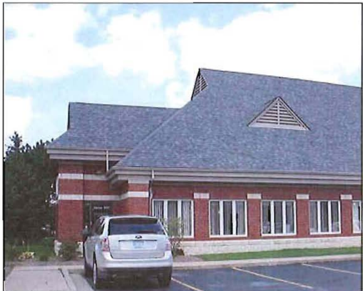
Figure 21 - Example office with single family residential character (ADCO Office Building 2009).
