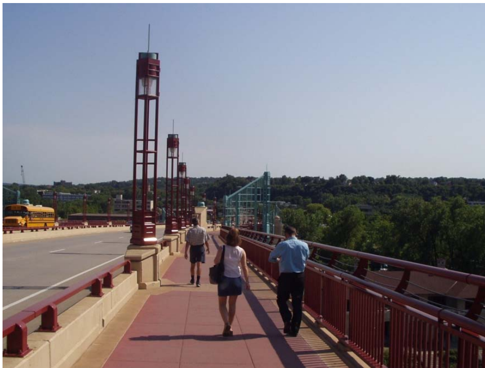
Wabasha Street Bridge in St. Paul Minneapolis
