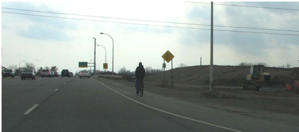
Existing conditions for the Novi Street overpass
