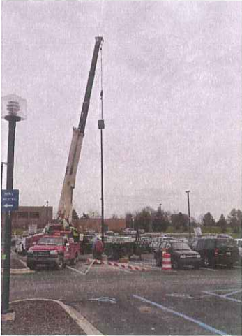
Civic Center Lighting Pole Installation
