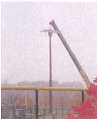
Installation of Power Park Lighting
