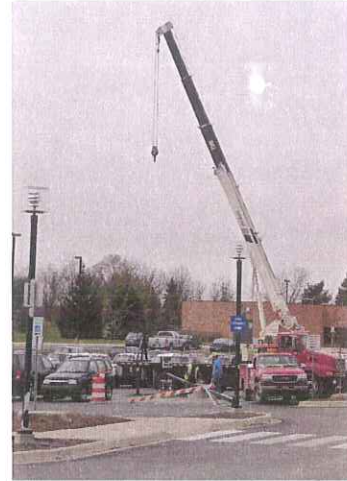
Civic Center Lighting Pole Installation
