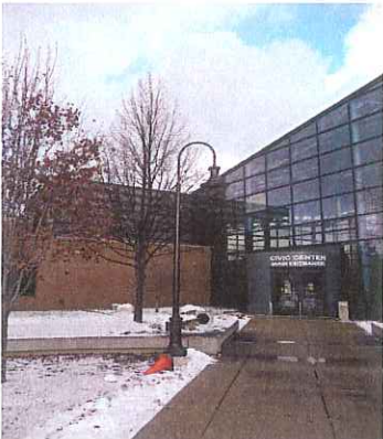
Pedestrian lighting at City Hall
