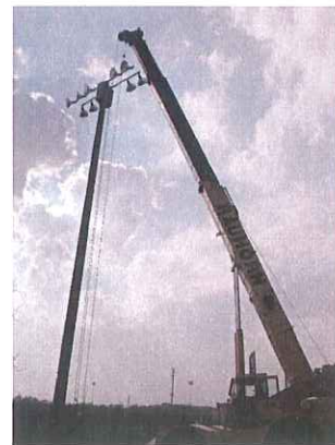
Power Park Lighting Installation
