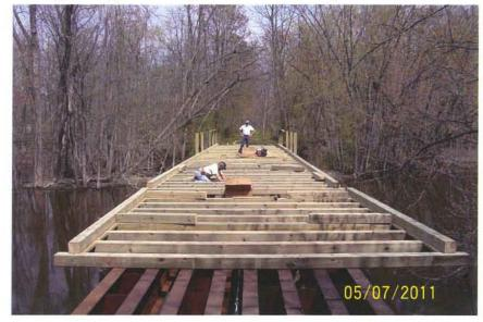
into trail between the Villages of Nashville and Vermontville in Eaton County. Project included inspection of old bridge and development of deck details that could be built by vocational education class at the Maple Valley High School. To provide 14 foot clear width, the deck is designed to cantilever out from existing steel beams of railroad structure. Construction in the spring of 2011.
