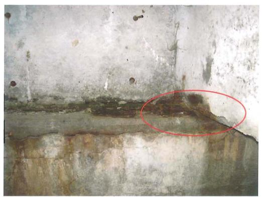
Typical condition of bearings. Bearings have heavy pack rust and section loss. Concrete at bottom of beam at bearings is cracked.
