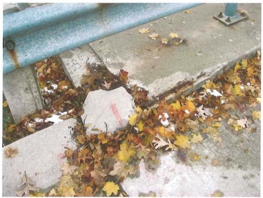
Toe of west sidewalk and top of abutment wall – spalled concrete with exposed reinforcement.
