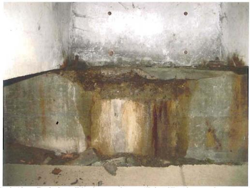
North Abut. Typical condition between beams 4E thru 8E. Abutment is wet, seat is spalled and rust stained.
