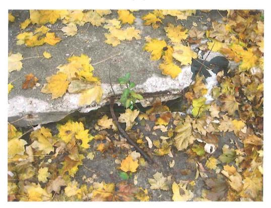
Toe of west sidewalk – spalled concrete, expose and corroded reinforcing steel.
