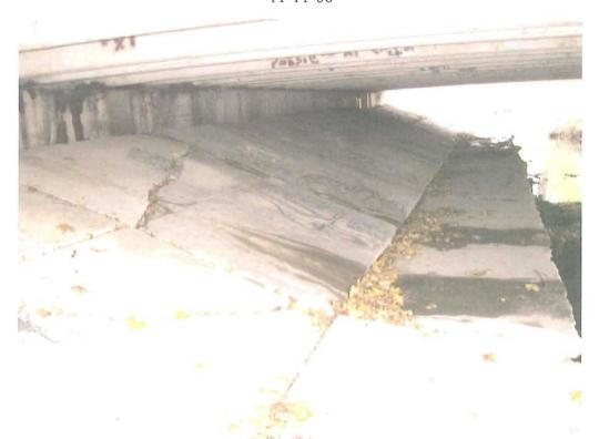
North abutment and slope protection. Slope paving is undermined, settled, and cracked throughout.
