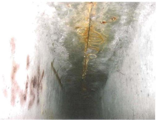
Typical condition of joints between beams – Top flange is wet with efflorescence and rust staining.
