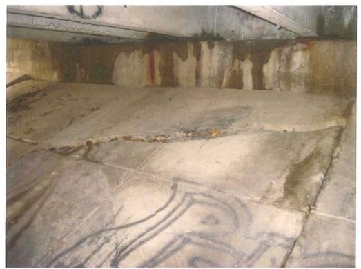
North Abut. Seat below beams 3W-6W wet. Beam seat is spalled between beams with exposed rebar. Spalls extend under bearing areas approx. 5%.
