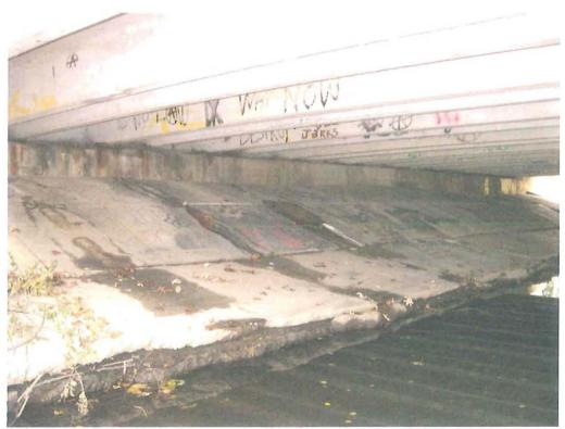
South abutment and slope protection. Slope paving is undermined, settled, and cracked throughout.
