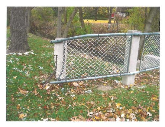
Damaged concrete post in the northeast quadrant of the bridge.
