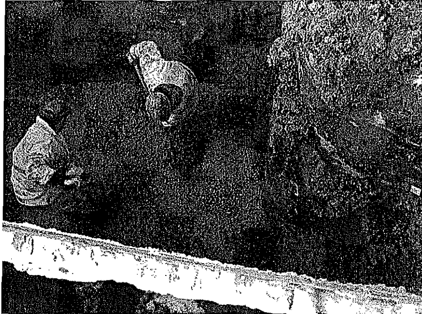
Placing new pipe out of the existing sanitary manhole. Stone bedding and backfill over the pipe.
