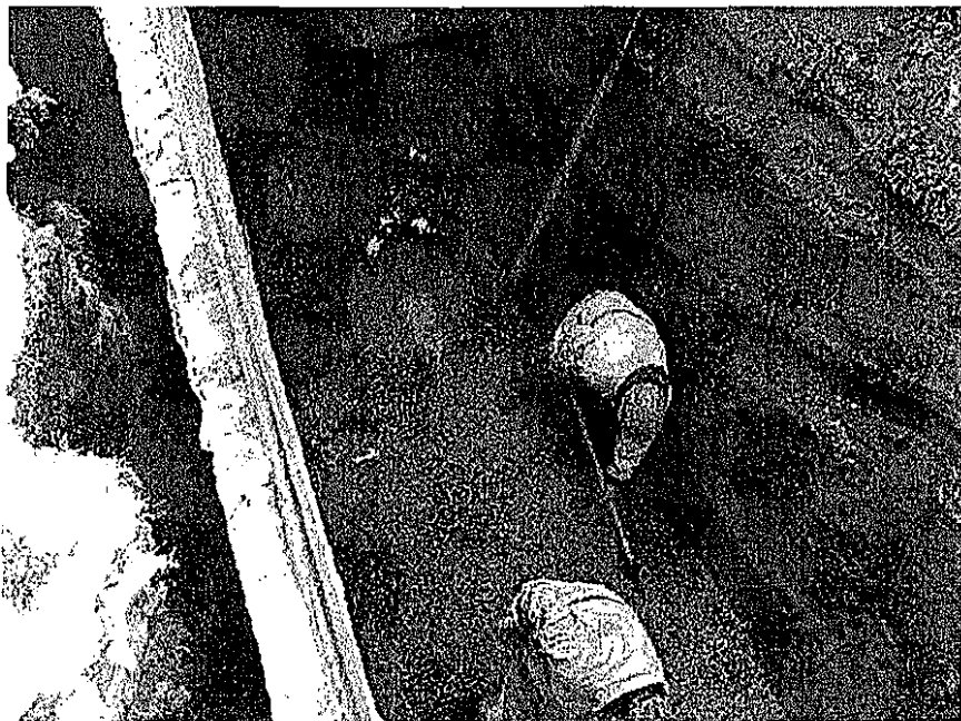
Placing new pipe out of the existing sanitary manhole. Stone bedding and backfill over the pipe.
