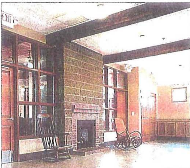
Modern construction materials like split-faced block and hollow metal door frames were combined with non-structural exposed wood beams and antique rockers to create a timeless feel for the Visitors Center.
