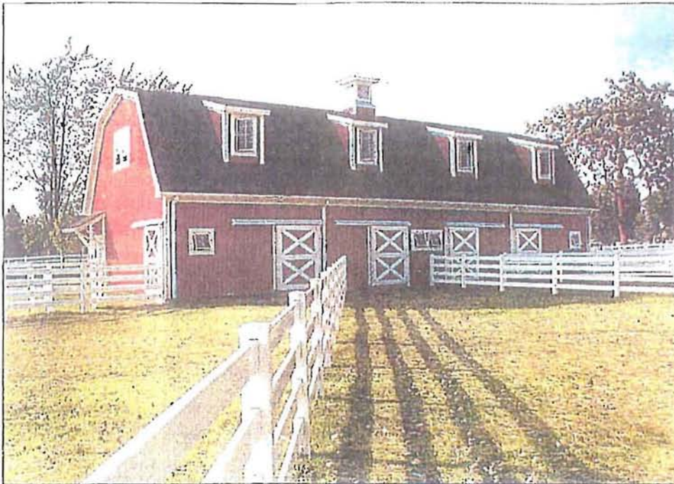
Each stall in the barn provides access to a pie-shaped paddock. The paddocks are separated with PVC fencing because the arsenic content in Wolmanized™ wood makes it hazardous for animals to chew on.
