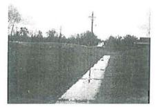
Draining west, existing paved ditch adds to steep slope issues upon road widening.
