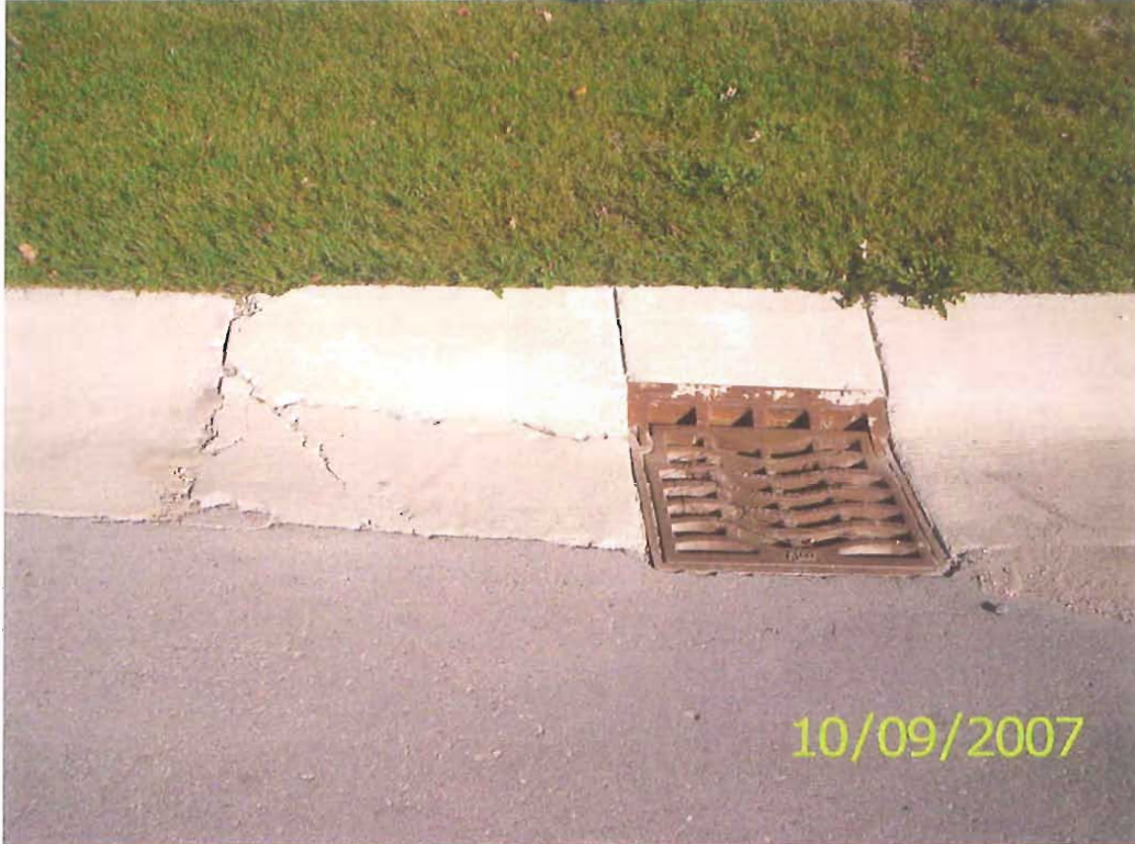
Here are some of the locations where the curb and gutter is cracked.
