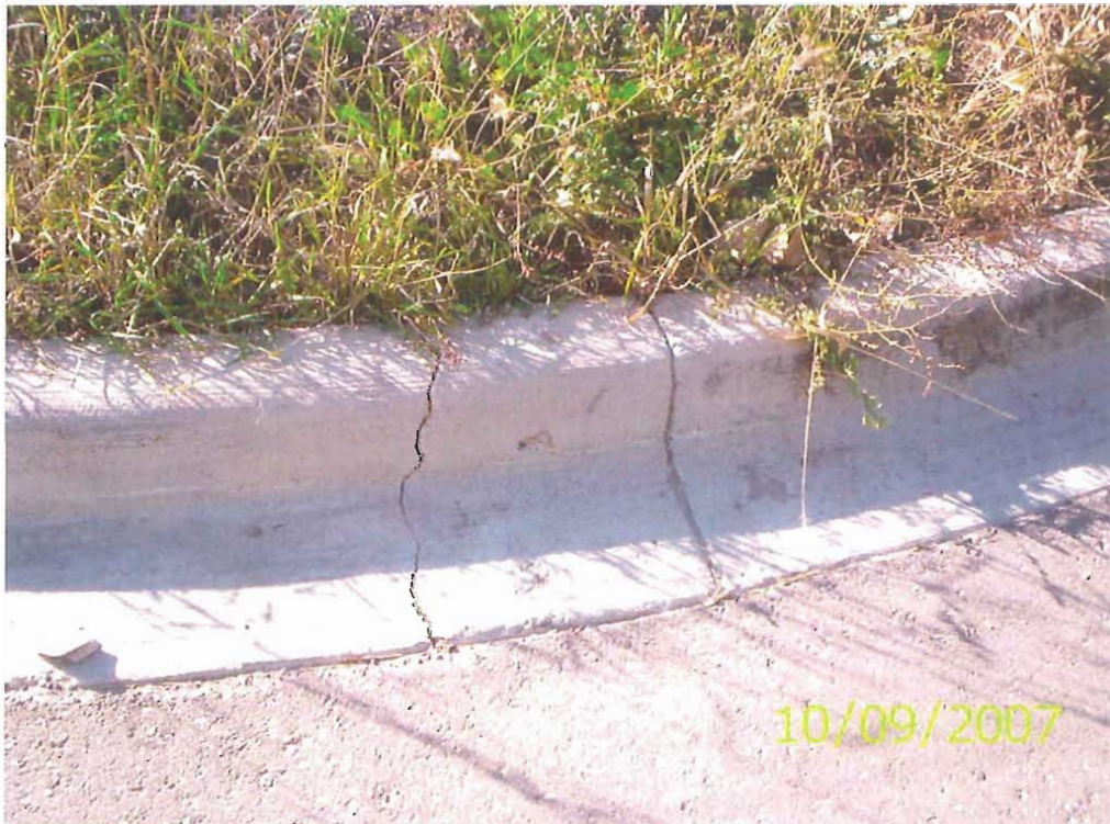
Here are some of the locations where the curb and gutter is cracked.
