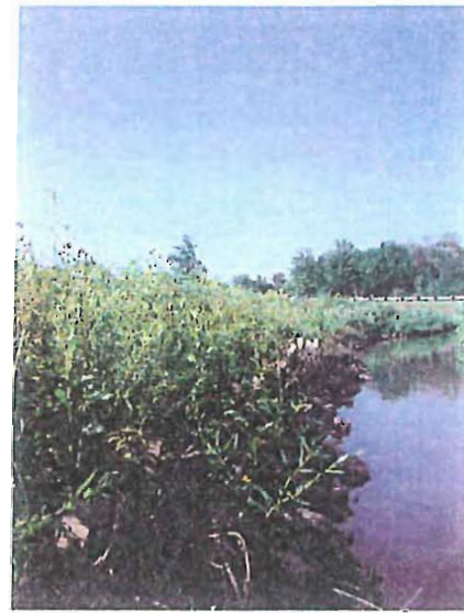
Photo 15: Gibson Drain streambank stabilization (Sterling Heights, MI)
