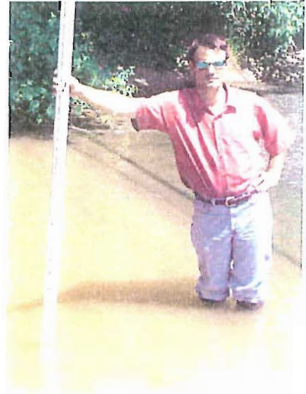
Photo 10: Streambed is 1-2 feet below apron
