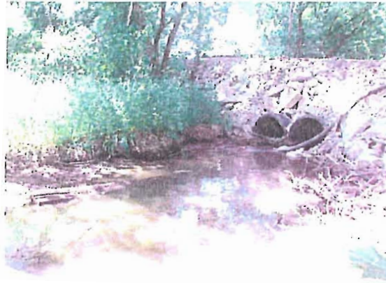
Photo 21: Possible location for sediment trap
