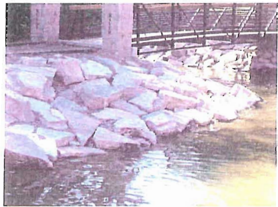
Photo 8: Example of riprap protection (Quarton Lake, Birmingham, MI)
