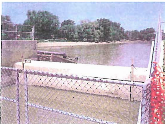
Photo 3: Existing Meadowbrook Lake Dam spillway
