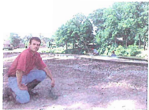
Photo 6: Installed Pyramat spillway (Quarton Lake Dam)
