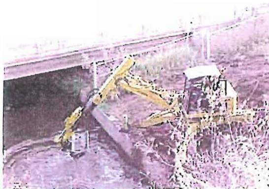
Photo 20: Cleanout of a sediment trap (Duluth, MN)
