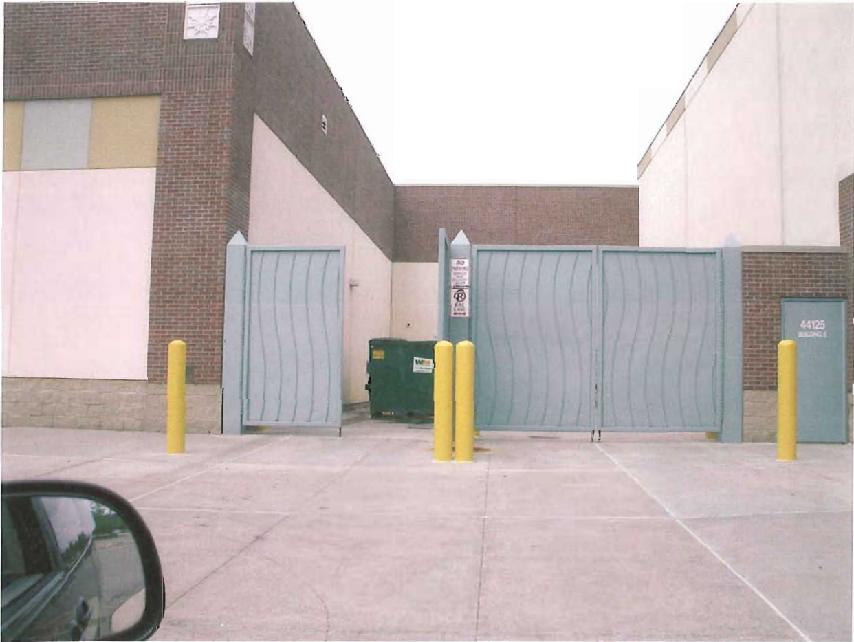
Existing Northeast Dumpster Enclosure/Loading Area
