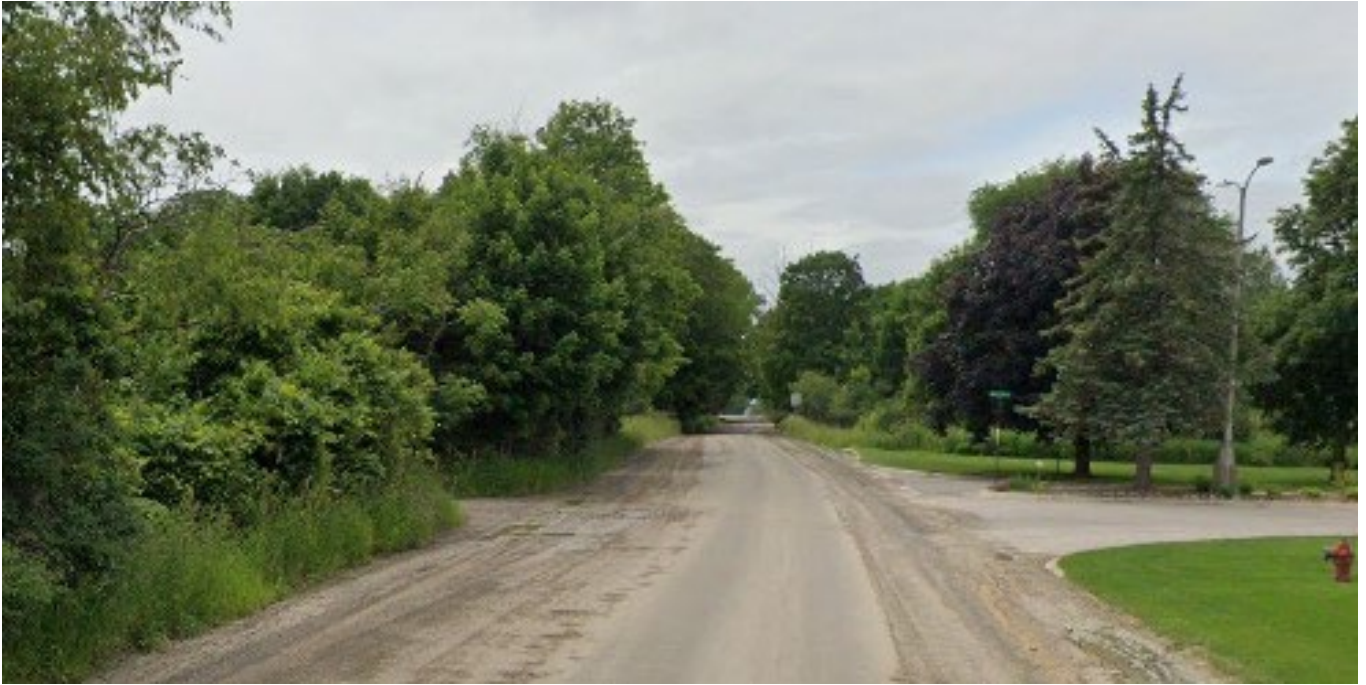
Before – 12 Mile east of Catholic Central entrance, looking west.
