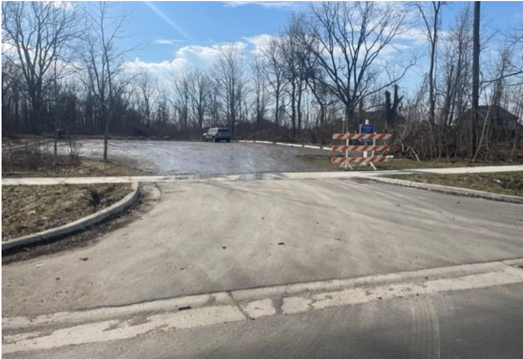
After – NW Park parking lot, looking south from 12 Mile Road
