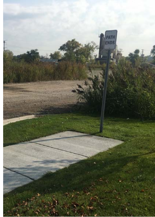
End of segment; possible extension in future
