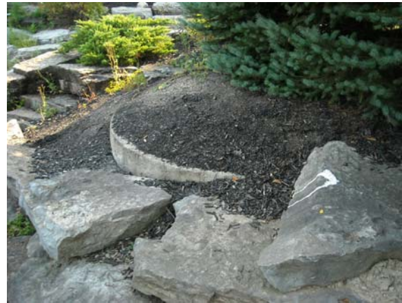
Structure surrounded by Landscaping
