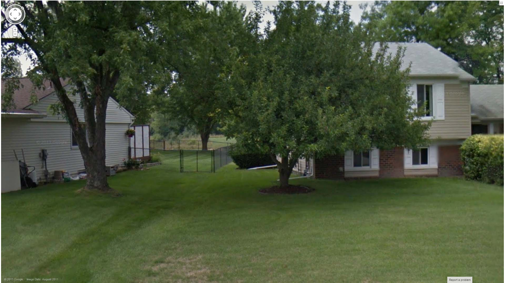
Access to Structure #10
