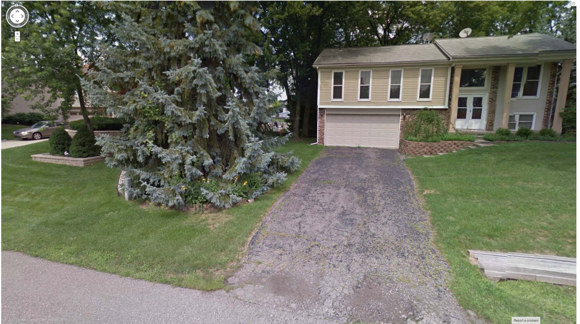
Access to Structure #5
