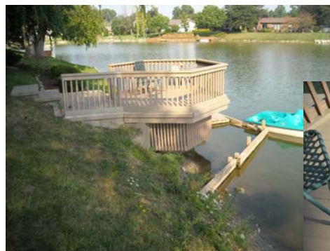
Deck built over Structure
