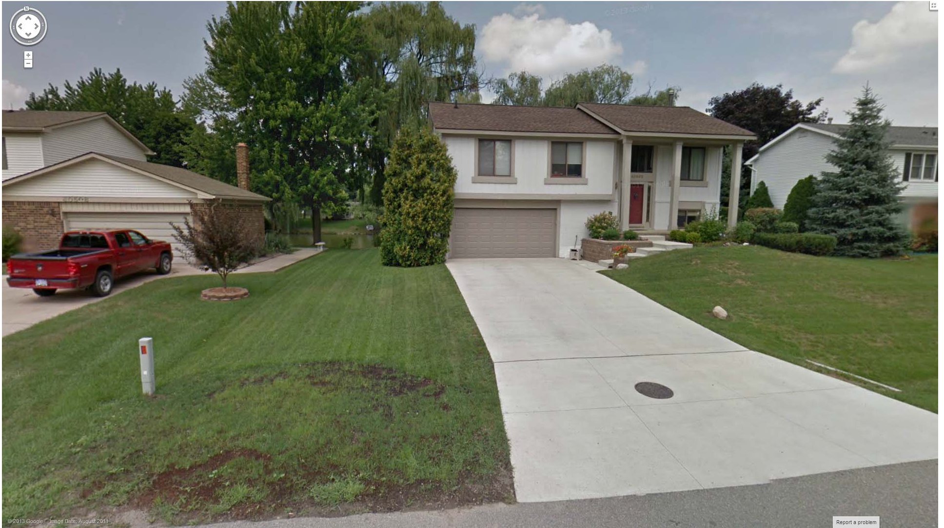
Access to Structure #4
