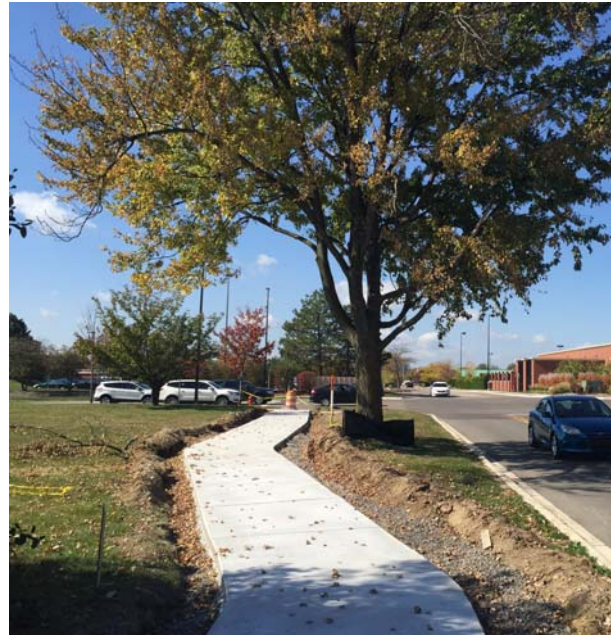
Sidewalk under construction in Town Center Area
