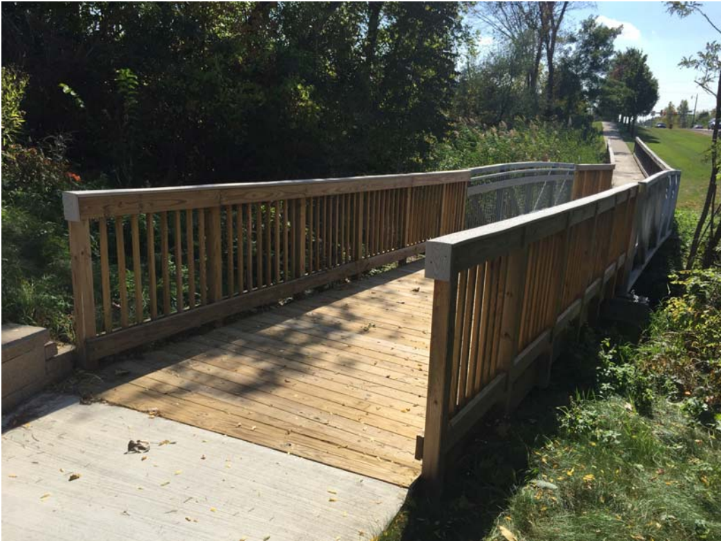
Sidewalk along Meadowbrook between Eleven Mile and Grand Rive Avenue
