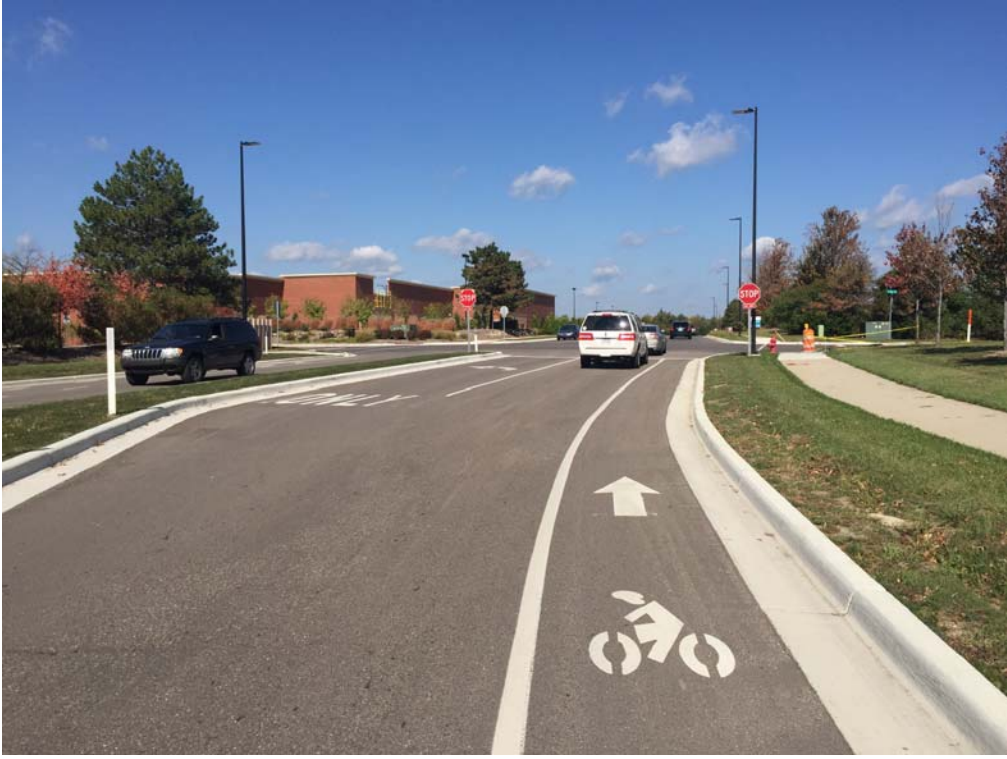
Town Center Drive Reconstruction with Bike Lanes
