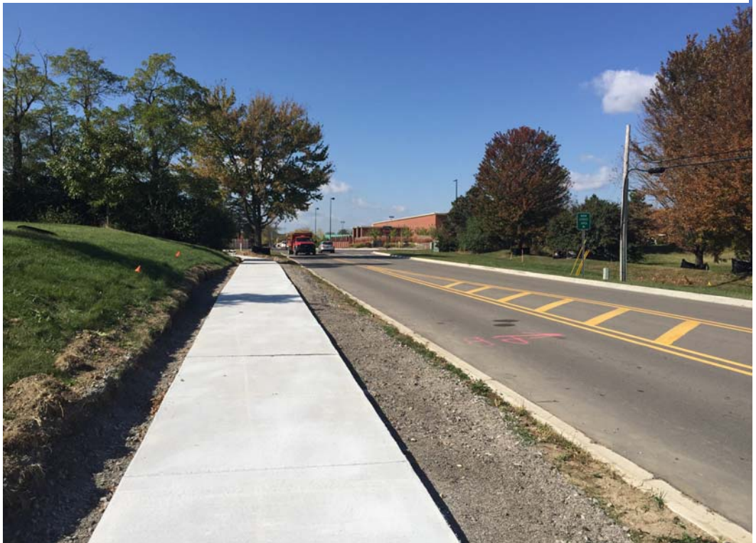
Pedestrian improvements around Novi Dog Park
