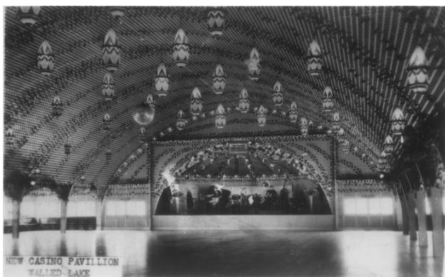
Figure 3: Interior of former casino/dance hall
